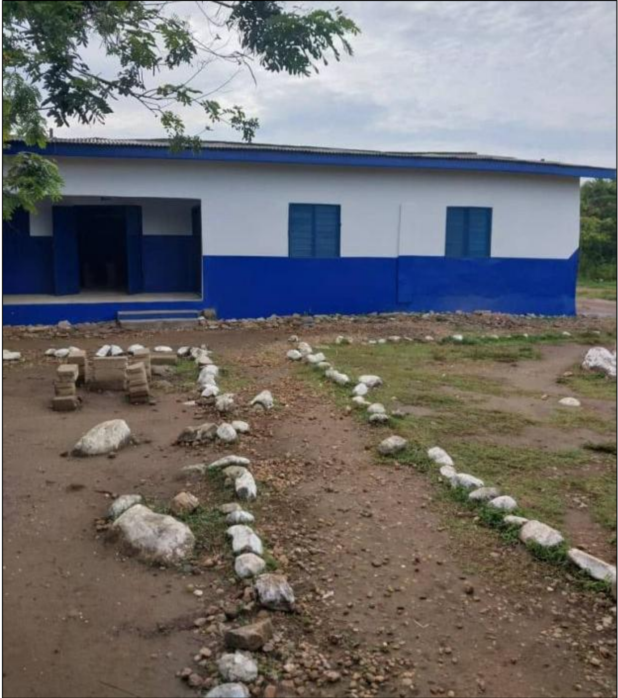
The exterior of the Winneba Anglican Primary School in Ghana after a renovation was completed thanks to more than $10,000 donated by retired UMass Lowell professor Jesse Heines. (Courtesy Jesse Heines)
